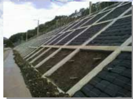
Reinforcement of existing slopes!
