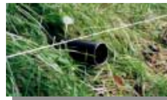
Improvement of drainage system and embankment stability!
